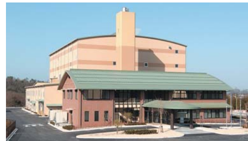
Eco Slag Center at Tottori Prefecture's Greater Western Area Administrative Management Union
