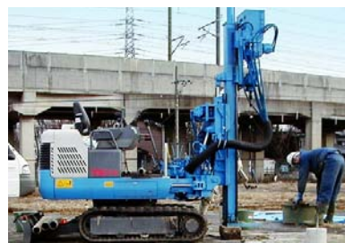
Extracting a sample with a simple boring machine
