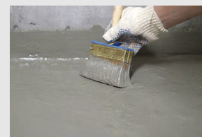
Waterproofing and anticorrosion paints
