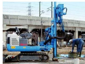
Extracting a sample with a simple boring machine
